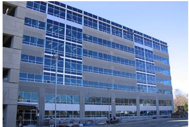
More than 165 FlexiDome cameras provide surveillance at Middlesex County Court.
